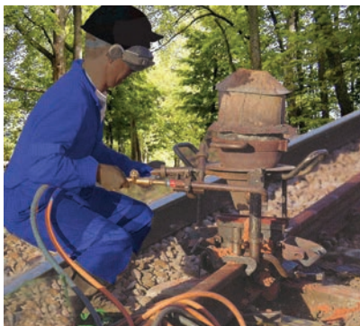
Figure 3.11 Thermit process for joining railway tracks
